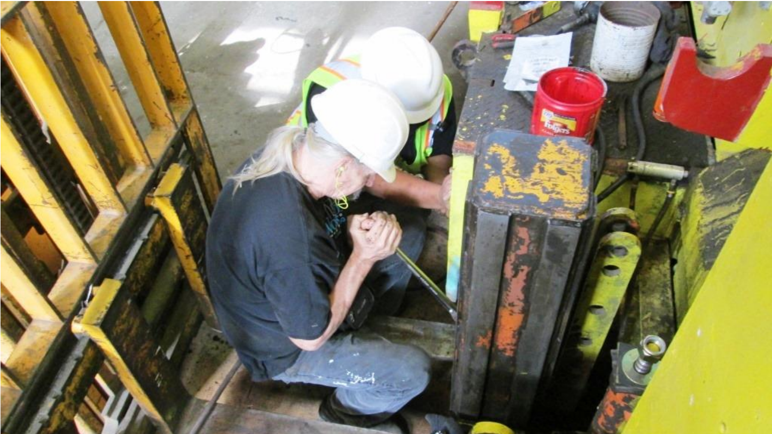
Fred and Anthony tighten-down new specialized bolts on the regulator
