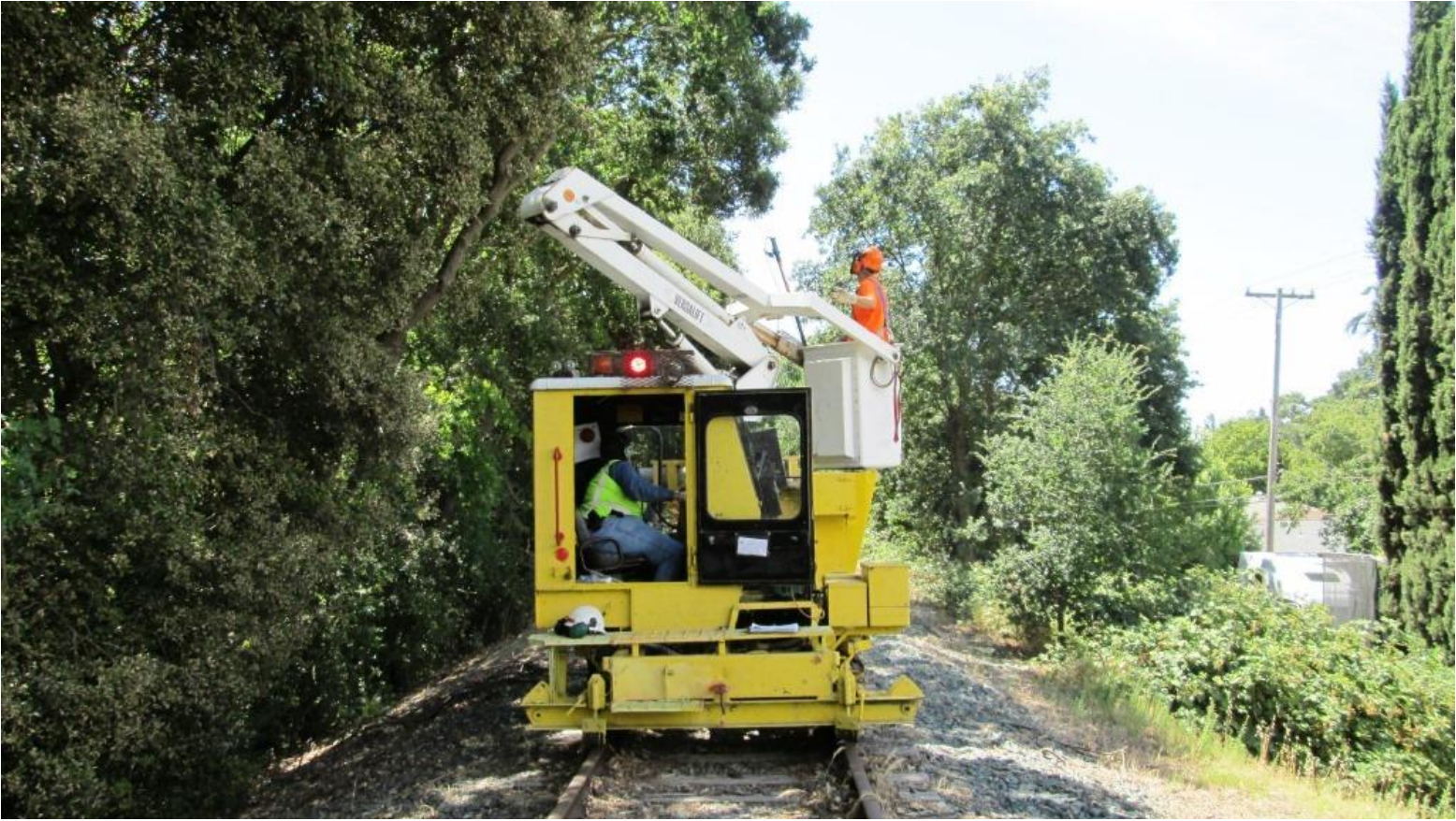
Heather operating the man-lift chauffeurs Dave further down the line
