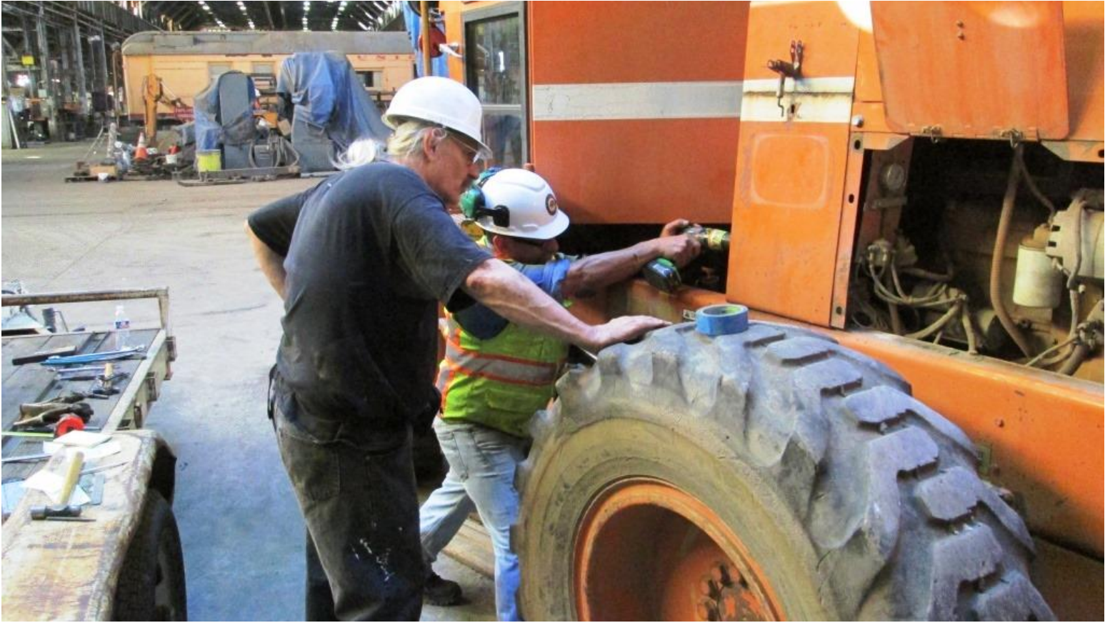
Joe and Fred drilling a new hole in the engine compartment casing on the loader for the installation of a new battery switch
