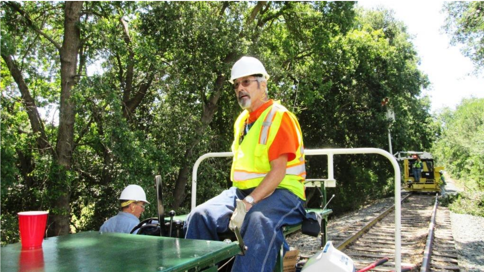
Ed piloting the A-6 motorcar keeps it close – but not too close – to the man-lift
